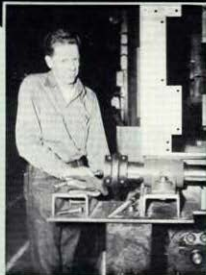
James Bishop, Steel Shop, has been here since June, 1951. Previously he had been employed by Studebaker. Jim is an Assembler. In this picture we see him working on a Sparkoff Cabinet for cleaning box car wheels. This machine will go to Almirante S. A., Buenos Aires, Argentina, South America. Jim is married and has three children. His chief interests are TV and all the sports.
